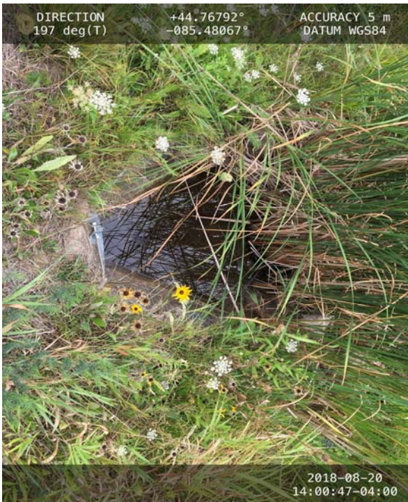
Photo 10: Basin # 1 swale inlet structure
